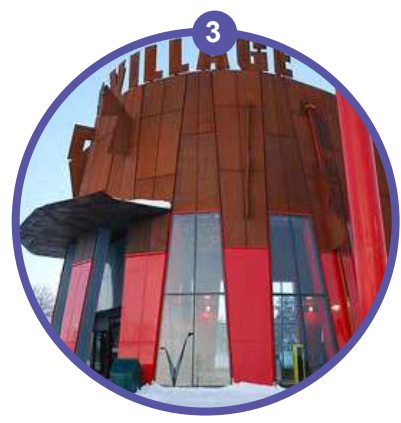
3 Pioneer Village Subway Station
